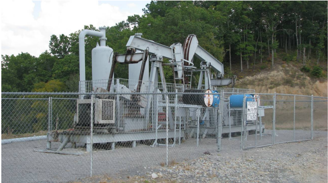
Figure 6-1. Pinnacle 97 Well Pad.
