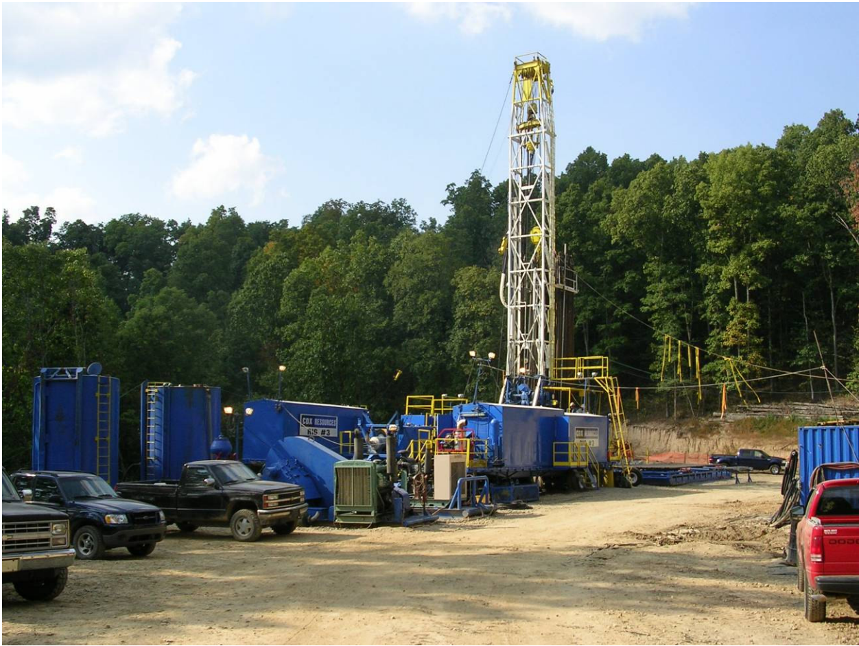
Figure 6-9. CDX Rotary Drill Rig
