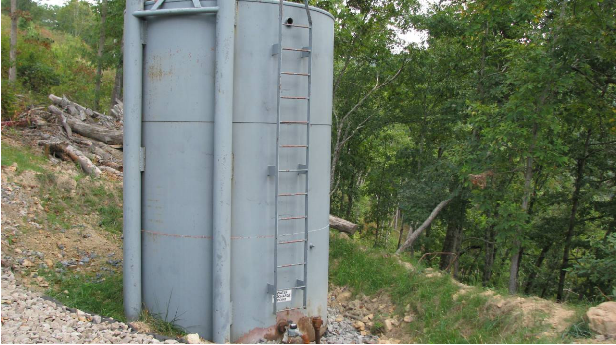
Figure 6-6. Wastewater Storage Tank
