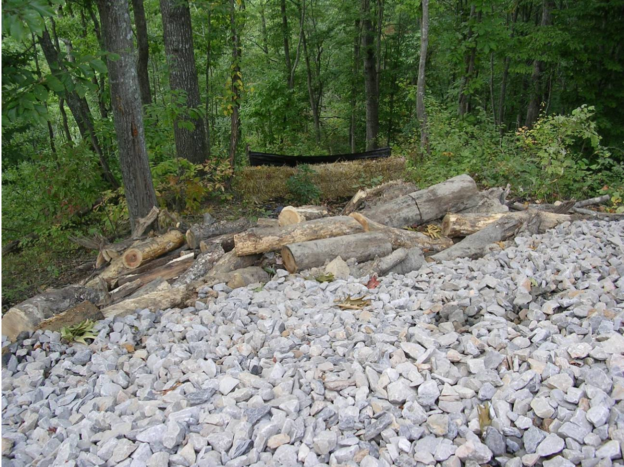
Figure 6-8. Gravel Apron and Hay Bails
