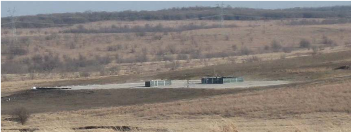
Figure 5.2. Gas well site on modified hillslope.
