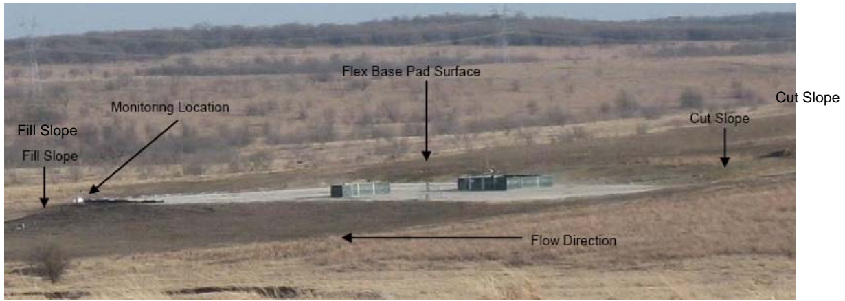
Figure 3.1. Gas well pad surface (GW1) on modified hillslope.
