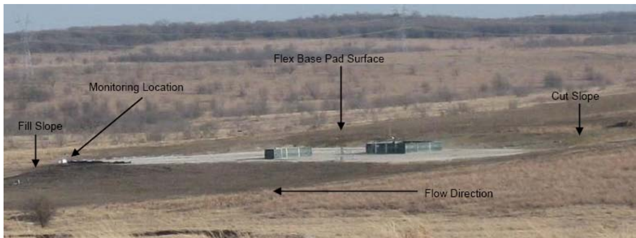
Figure 2.2. Gas well pad (Site 2) on modified hillslope.
