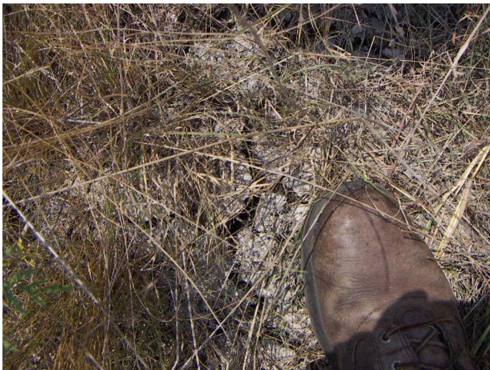
Figure 4.2. Cracks in the soil at the reference site.
