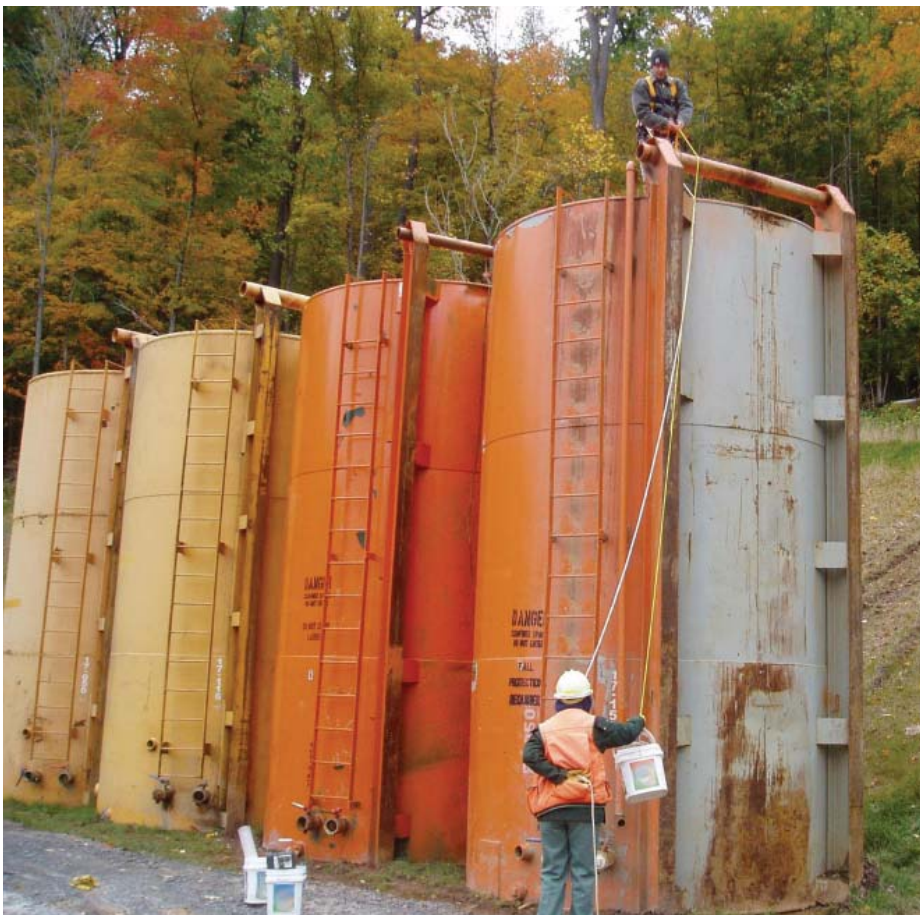
Figure 1.—The tank on the right is the one from which the flowback was sampled following refracturing of well B-800 on the Fernow Experimental Forest. The access inlet is on the top of the tank between the top of the ladder and the person preparing for sampling. The valves for emptying or sampling fluid are located near the base of the ladder; there are two valves on each of these tanks and they are visible on the second tank from the right, just above the buckets on the ground. Photo by William Wilson, U.S. Forest Service.
