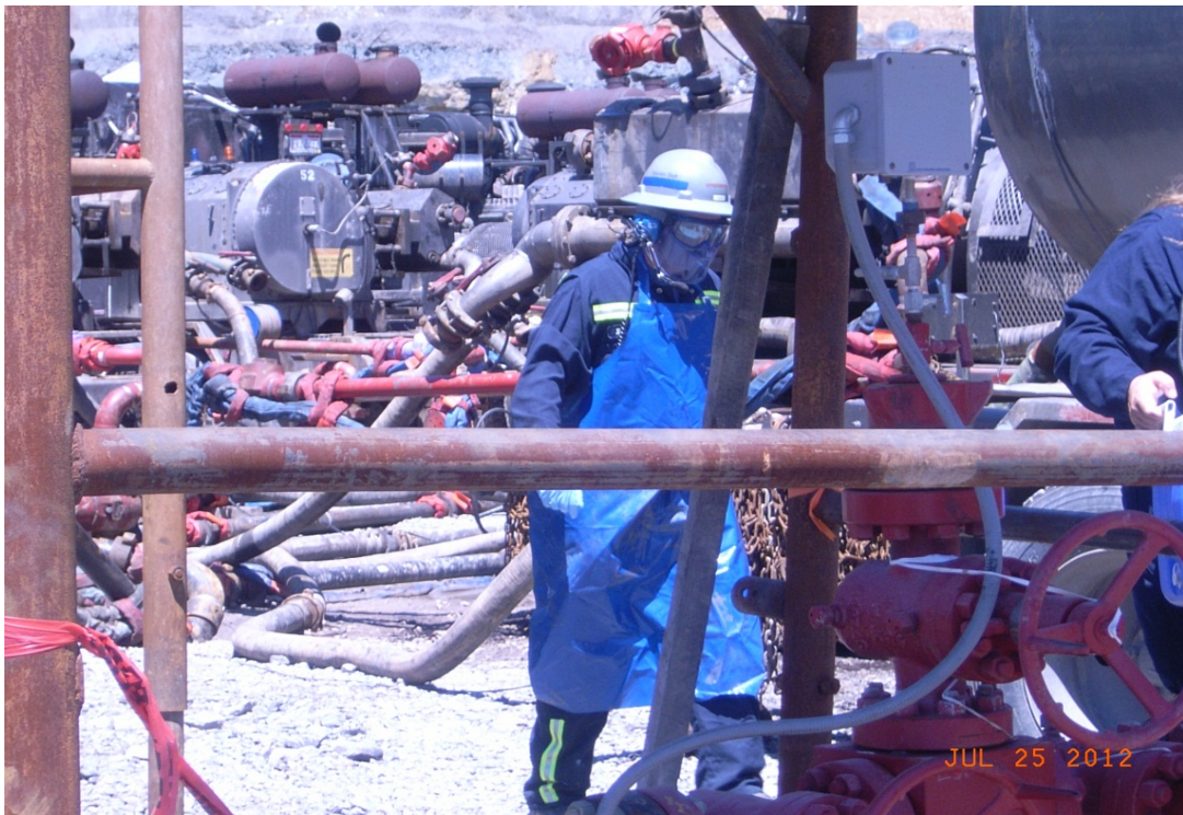
Figure 9: Sampling Hydraulic Fracturing Fluids and Water Mixture before Entering Well
