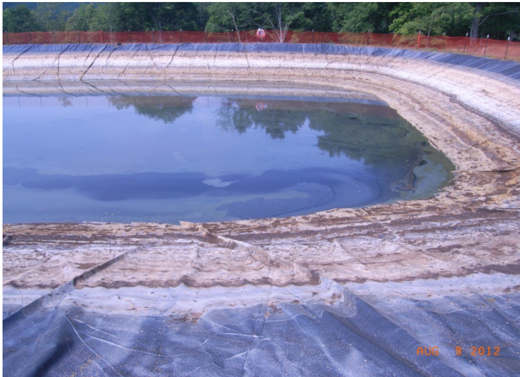
Figure 12: Composite Flowback Stream Sample at Donna Pad Single-Lined Pit
