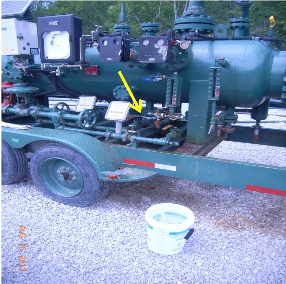
Figure 13: Weekley Pad Sample Area – Sample taken from the nozzle (see arrow)
